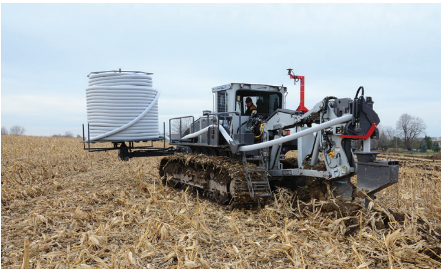
SPECIALIZED AGRICULTURAL TILING EQUIPMENT USES GPS TECHNOLOGY TO ENSURE ACCURATE INSTALLATION
